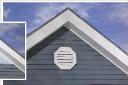
Gable Vent Cap installed with siding
