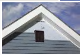
Gable Vent Base installed with siding
